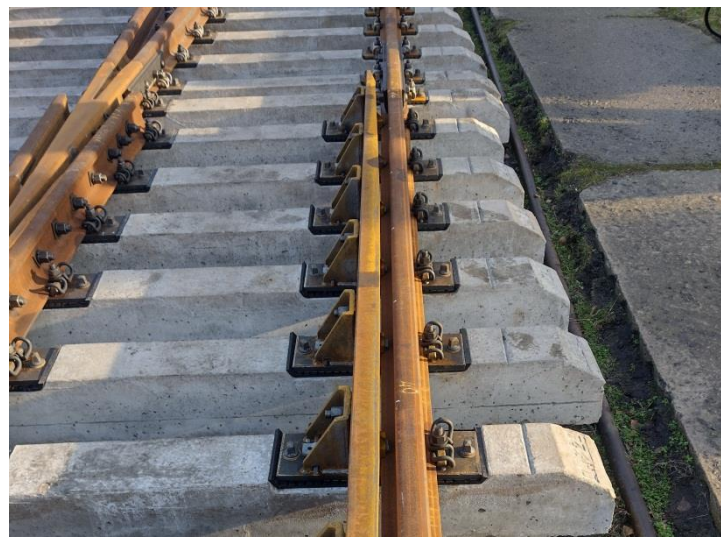
Figure 2. Frog with guard rail of a R65 switch, 1/11 crossing, track gauge 1 435 mm (Ukraine)
