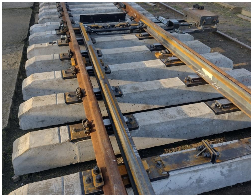
Figure 1. Switch points of a R65 turnout with a 1/11 crossing, track gauge 1 435 mm (Ukraine)
