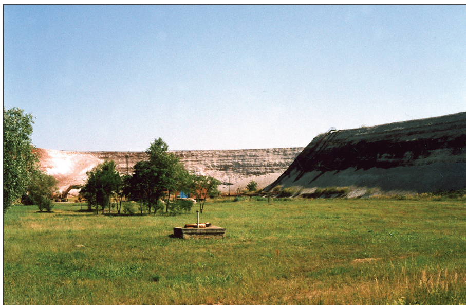
Photo 1. Observing wells monitoring water quality along the dam of red sludge reservoir (Photo by JUHÁSZ, Á. 2003)
