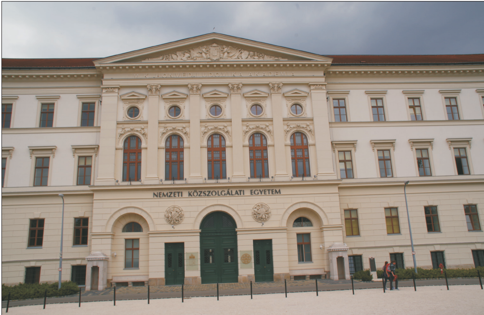
Photo 3. The new campus of the National University of Public Service accommodated in the 19 th century classicist building of a former military school (Photo by Boros, L.)
