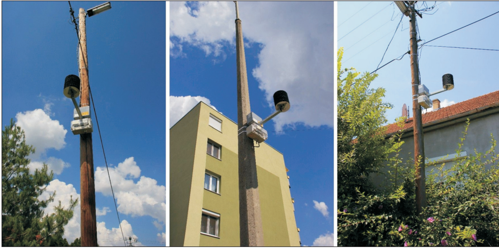
Photos 1–3. Typical setup of monitoring stations
