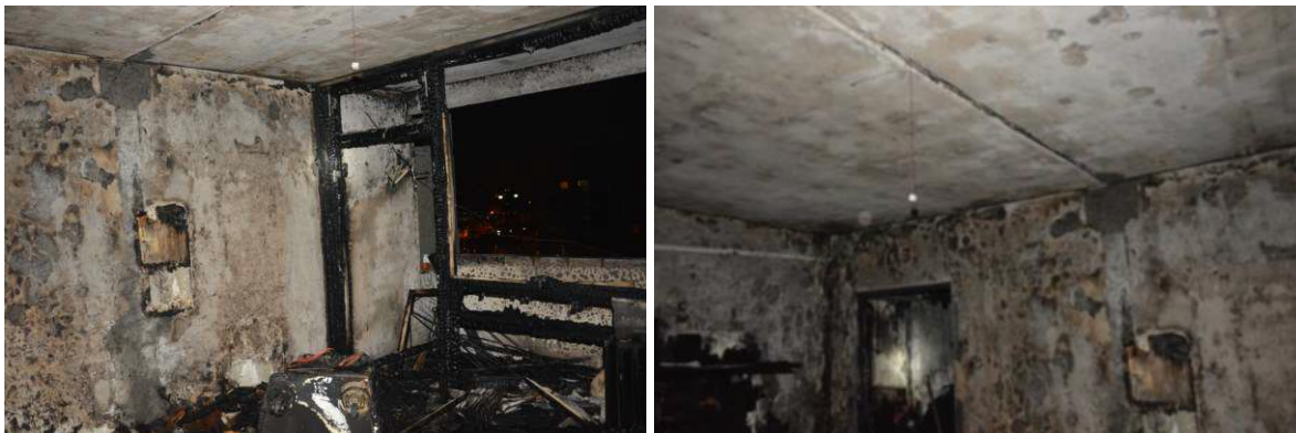
Figure 2. Location of a fire in a 9 th floor apartment of a panel residential building, 2020.
