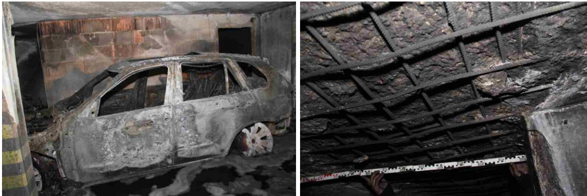
Figure 3. Fire scene of a car parked in an underground garage, 2017.
