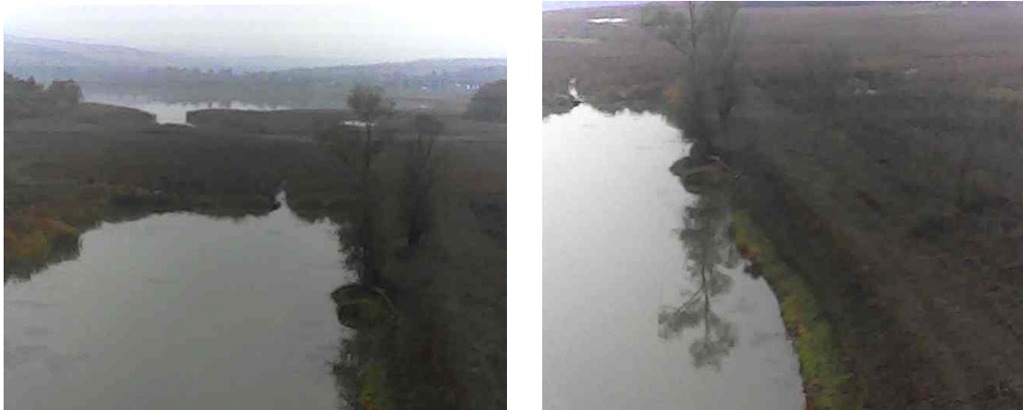
Figure 6 - Photo of the mudguard dam made to reduce the negative effect after heavy rain.
